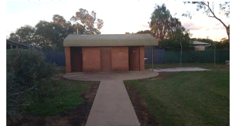
Toilet block (upgrades / accessible toilet in longer term)
