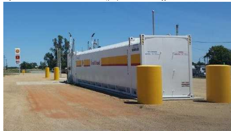
New Shell fuel station (south of rail line)
