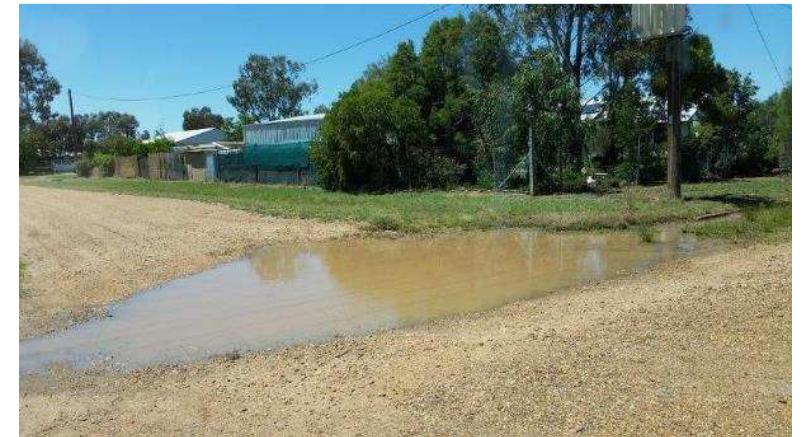
Cnr Clyde & Gunningbar Sts (drainage issues/extend gutter/review levels)
