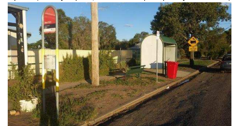
Mitchell Hwy outside Café (landscape upgrade/replace bin/fix kerb & gutter and road edge/widen footpath/accessible bus shelter & timetable)
