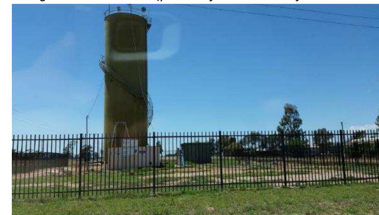
Nevertire water tank (repainting – re-roofing)
