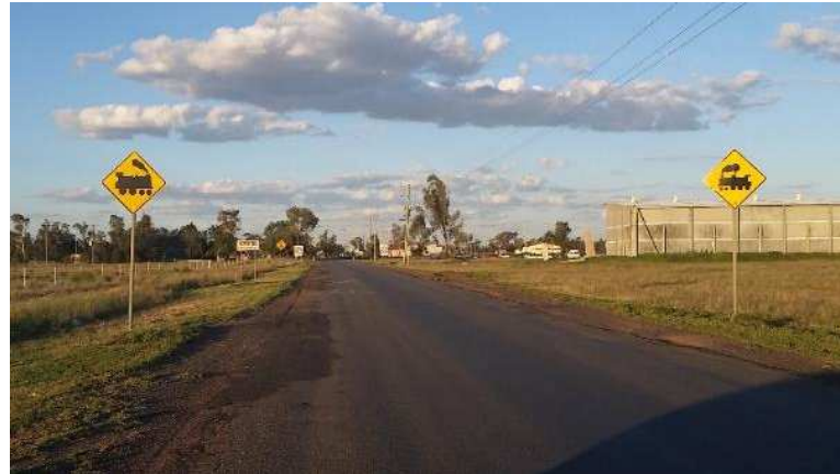
Road upgrades may be required in future due to increased usage
