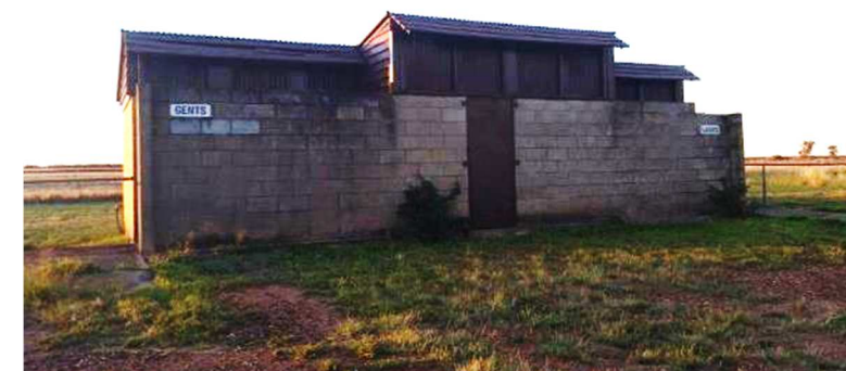
Discuss upgrades required to toilet block (especially if camping allowed)
