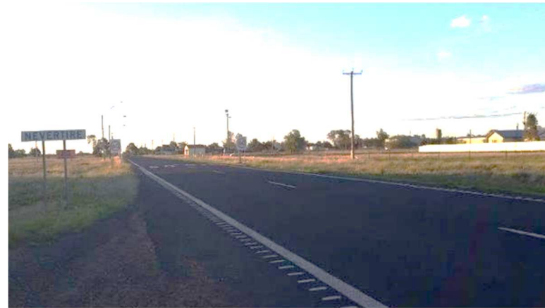
'Nevertire' black on white village signs & street lights (add Key Facilities signs and additional street trees to emphasis entrance to Nevertire)
