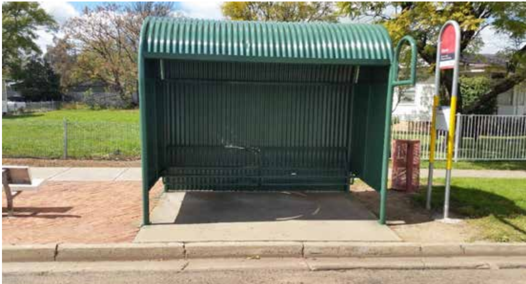
Photo 1. Existing Subject Bus Shelter
