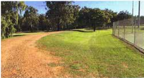
The existing levee bank south of Victoria Park Inner
